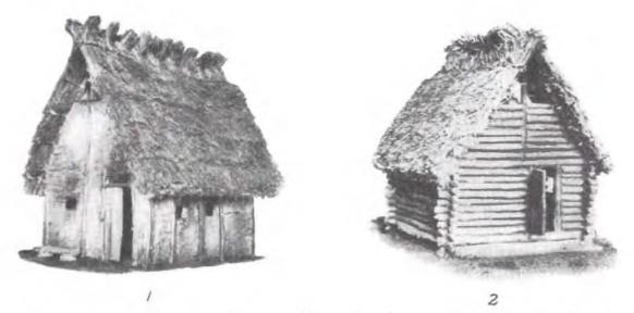
PLATE 59. Reconstructions of 1, a house with wattle and daub walls, and 2, a log cabin from the earlier village of Buchau, southwestern Germany. *After* Reinerth, 1936.
