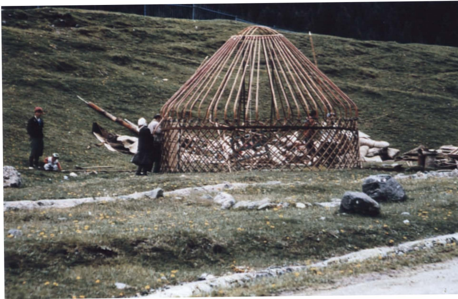
Figure 10. Erecting a framework for a ger , Xinjiang Uyghur Autonomous Region, June 1996. Photo: Emma C. Bunker
